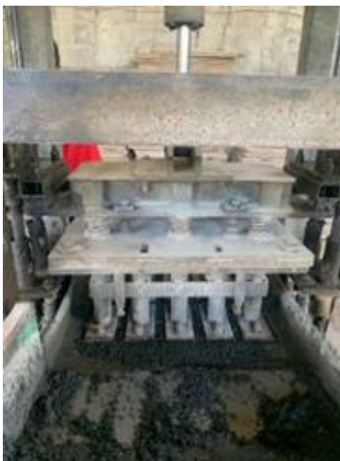
Gambar 3. Proses Pencetakan Paving Block
