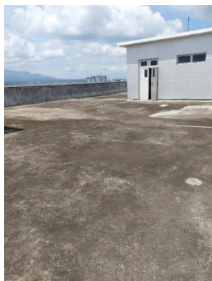
Gambar 1. Area Rooftop Gedung ICT UNDIP
