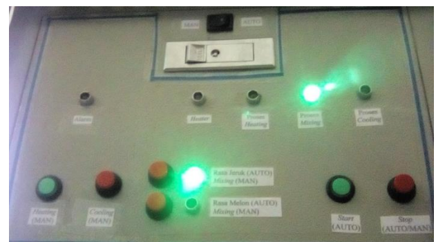
Gambar 10. Kondisi Panel Box Saat Proses Mixing
