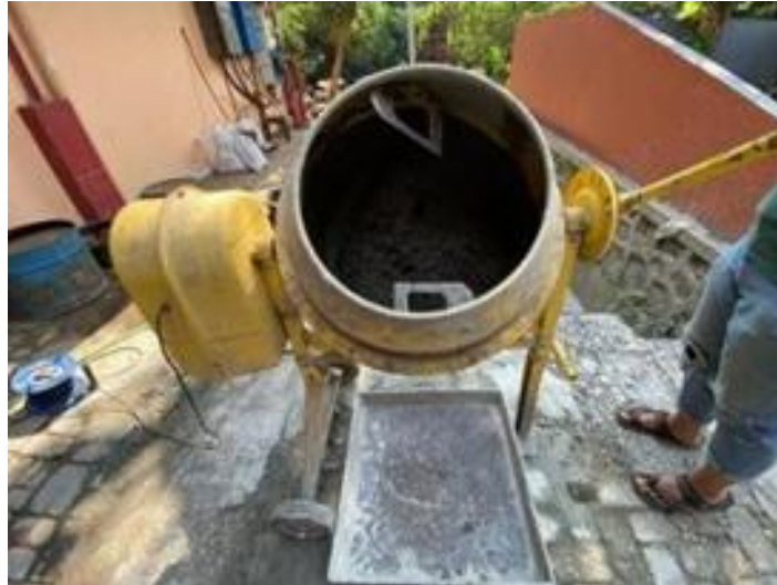
Gambar 3. Proses mixing beton
