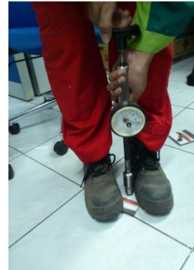
Gambar 9. Pengujian Pull-Off Test
