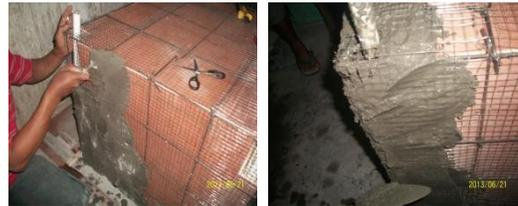
Gambar 6 Proses plester dinding ponton *ferrocement*
