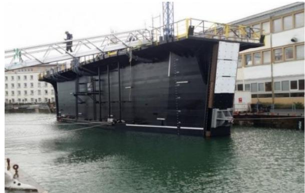
Gambar 1. Floating Caisson Gate
