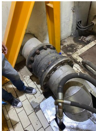
Gambar 1. Pompa Hydraulic Axial 500 LPS
