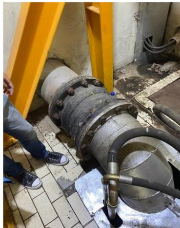
Gambar 1. Pompa Hydraulic Axial 1000 LPS
