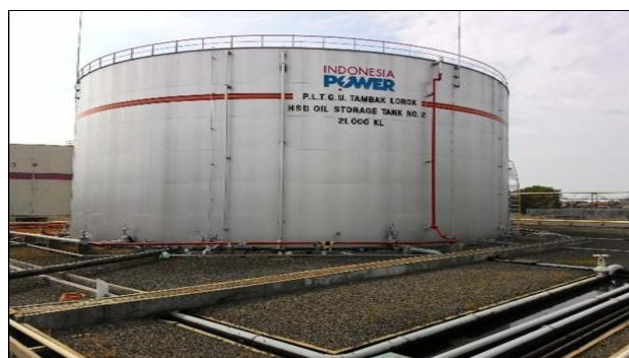
Gambar 1. HSD Oil Storage Tank
