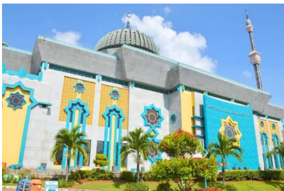
Gambar 5 : Jakarta Islamic Center (JIC) (sumber: http://duniamasjid.org/dunia_masjid/jakarta-islamic-center/ )
