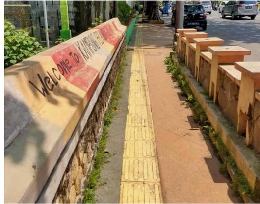
**Gambar 5.8.** Contoh paving taktil
