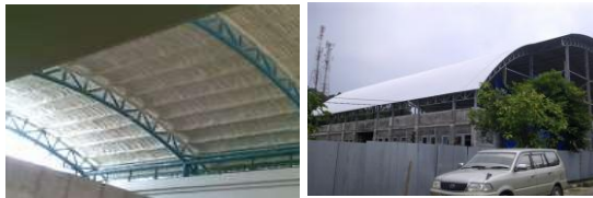
Gambar 32. Material atap – Spandex, Metal Aluminium Roofing Sumber : Penulis, 2012
