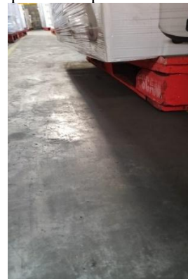
Gambar 4. Kondisi Warehouse Freezone 3
