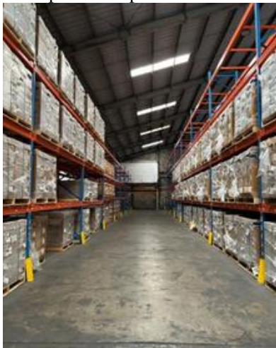
Gambar 7. Kondisi Warehouse Freezone 6
