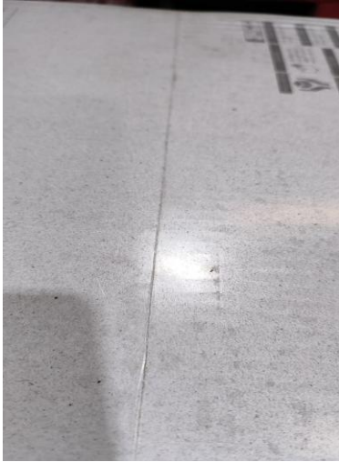
Gambar 6. Kondisi Warehouse Freezone 5
