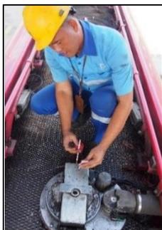
**Gambar 16.** Operator 8 Memasang Segel *Manhole Upper*
