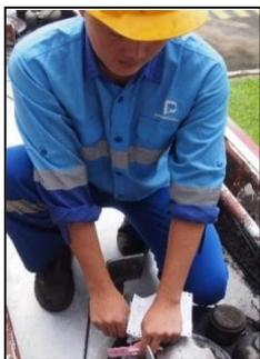
**Gambar 13.** Operator 5 Memasang Segel *Manhole Upper*
