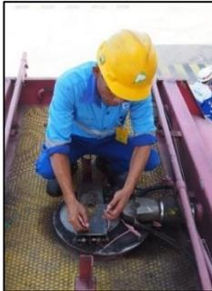
**Gambar 9.** Operator 1 Memasang Segel *Manhole Upper*
