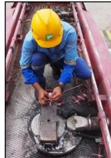
**Gambar 11.** Operator 3 Memasang Segel *Manhole Upper*
