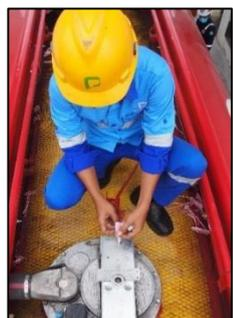
**Gambar 10.** Operator 2 Memasang Segel *Manhole Upper*
